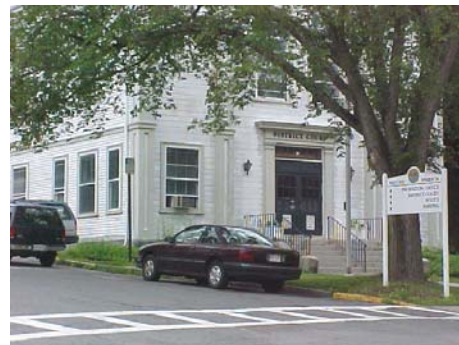
Exterior renovations to the former Town Hall/District Courthouse building respect the area's historic character.
