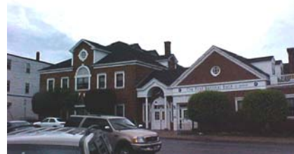
The above photos show the aesthetic improvements of removing overhead utility lines from Market Street.
